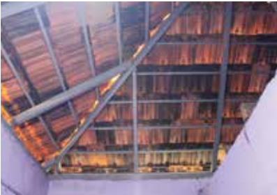
The truss work carried out for repairing of a damaged roof- another NITCAA project
